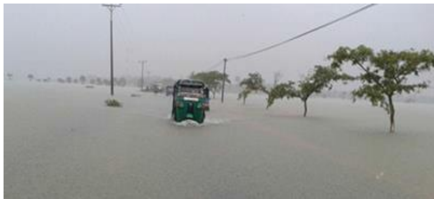
Figure 2. Flooding in 2019 - Location at (0+330 km)
