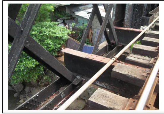
Figure 3: View of the cross girder-bottom girder connection
