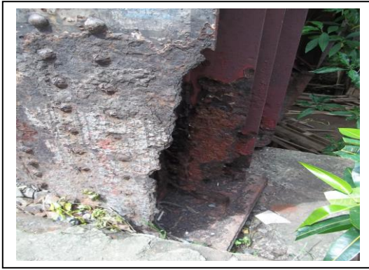
Figure 2: View of the corroded end box
